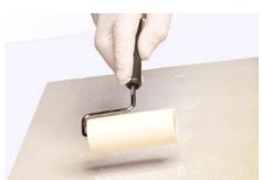
3. Apply adhesive using roller, spray or 2mm notched trowel.
