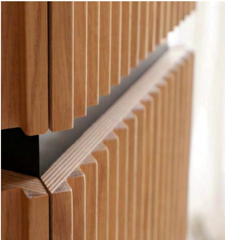
BIRCH PLYWOOD SUBSTRATE EXPOSED EDGES
